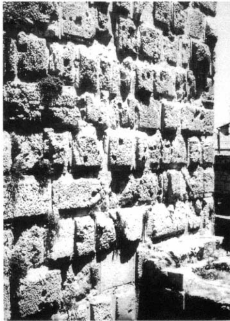
Fig. 28. Ashlar masonry with anathyrosis (Jerusalem, "Tower of David"). Photograph by Duane W. Roller.
