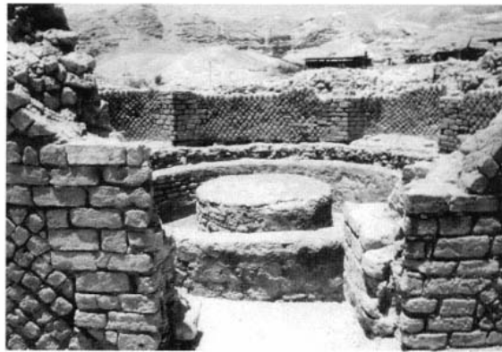
Fig. 27. Opus reticulatum in baths at second palace, Jericho. Courtesy Letitia K. Roller.
